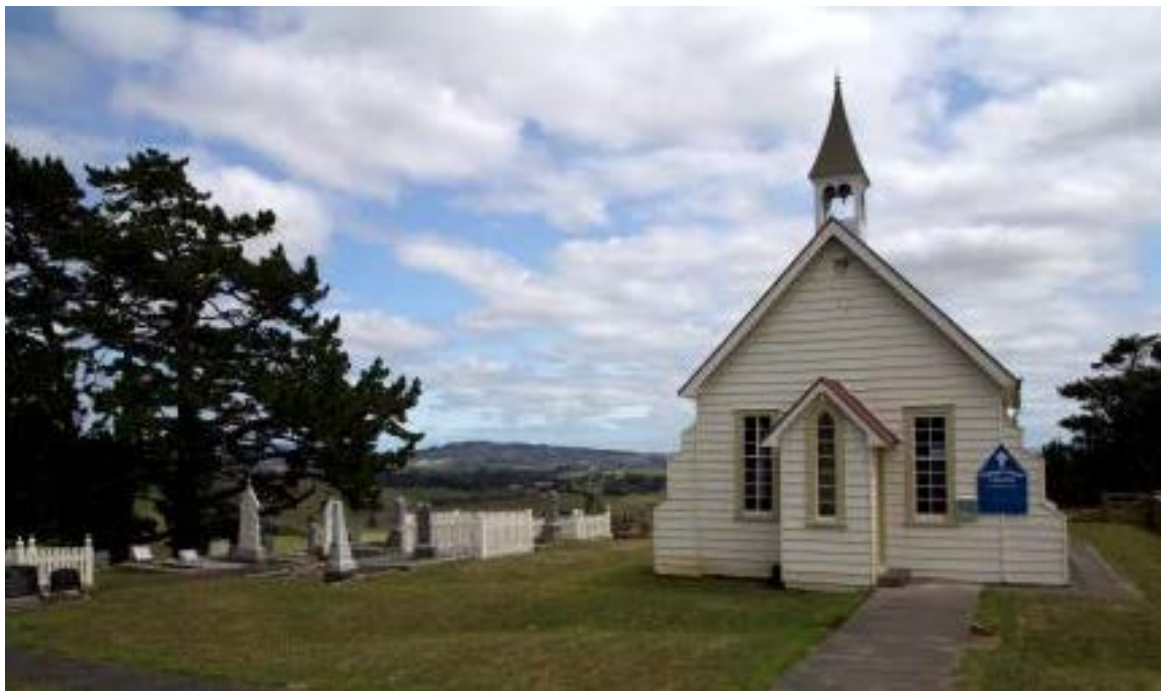
Figure 148. Pukekohe East Presbyterian Church today - front elevation and graves. Photo: AC, January 2014.
