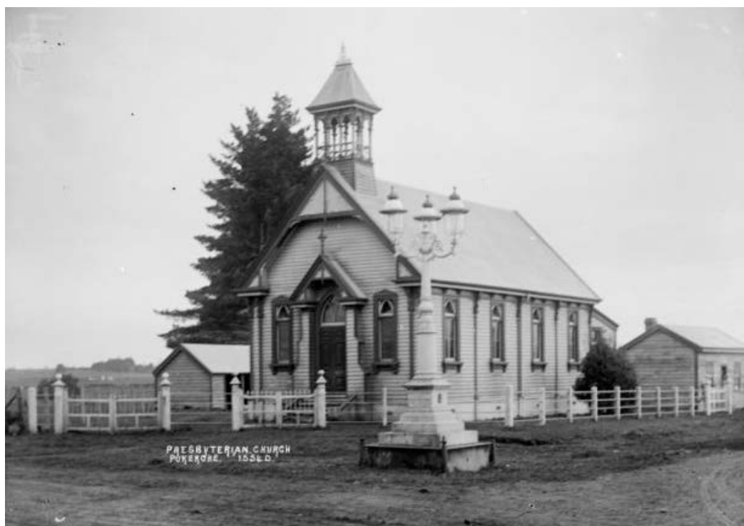
Figure 143. Pukekohe Presbyterian Church and outbuildings - corner of Queen and Seddon Streets c. 1915. ATL: 1/2-001335-G.
