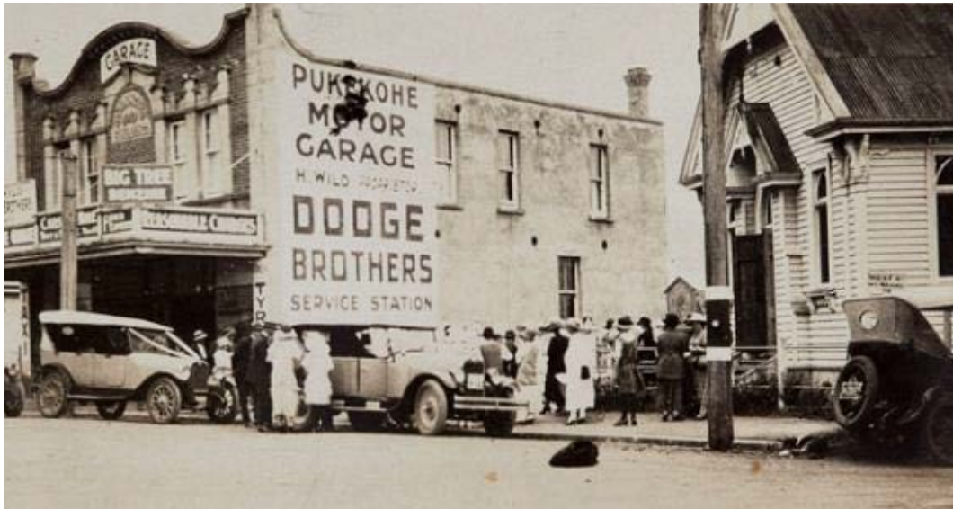
Figure 45. O'Connor's Building, West Street, 1924. Footprints 03237. Franklin Heritage Collection Pukekohe Library, Auckland Libraries.
