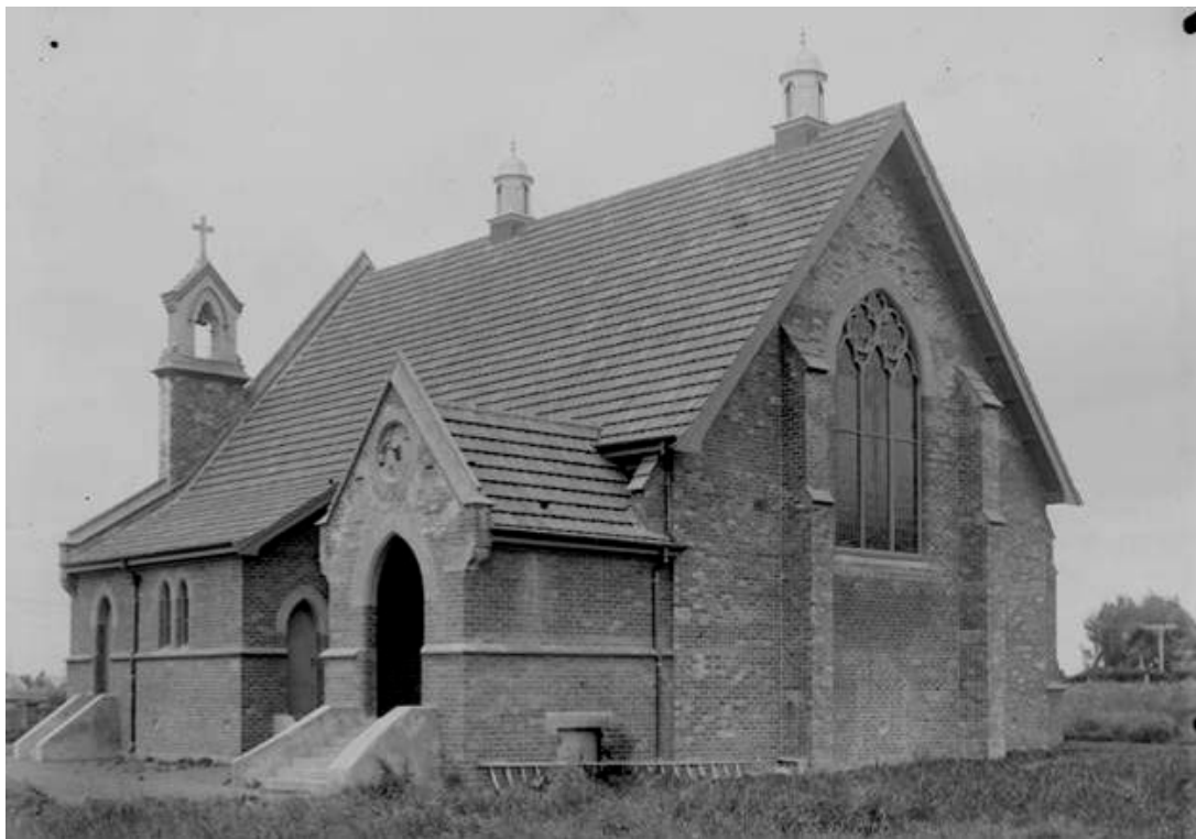
Figure 153. St Andrew's Church shortly after completion in November 1933. Sir George Grey Special Collections, Auckland Libraries, 4-6314.
