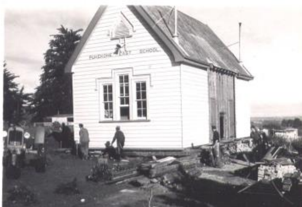
Figure 167. School building while being reorientated c.1947. Stone, C 2005.
