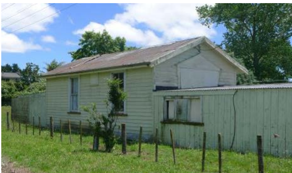
Figure 25 Suspected former police station associated building. Kauri Road. Eastern elevation. Photo: AC, December 2013.
