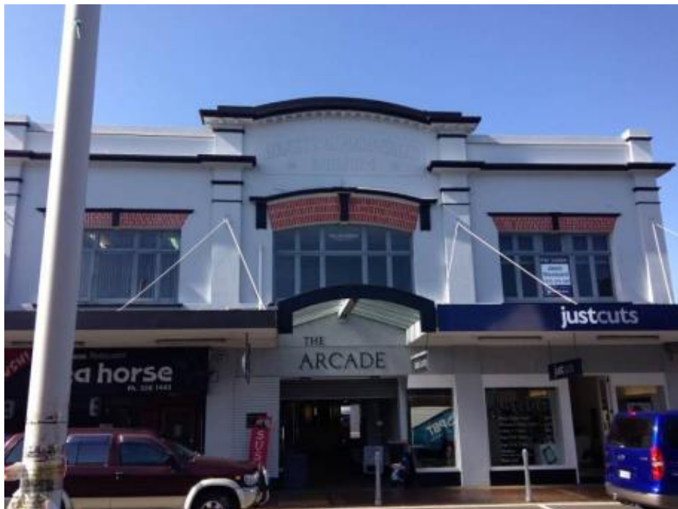
Figure 107. Beatty and Marshalls Building today, King Street. Photo: AC, January 2014.
