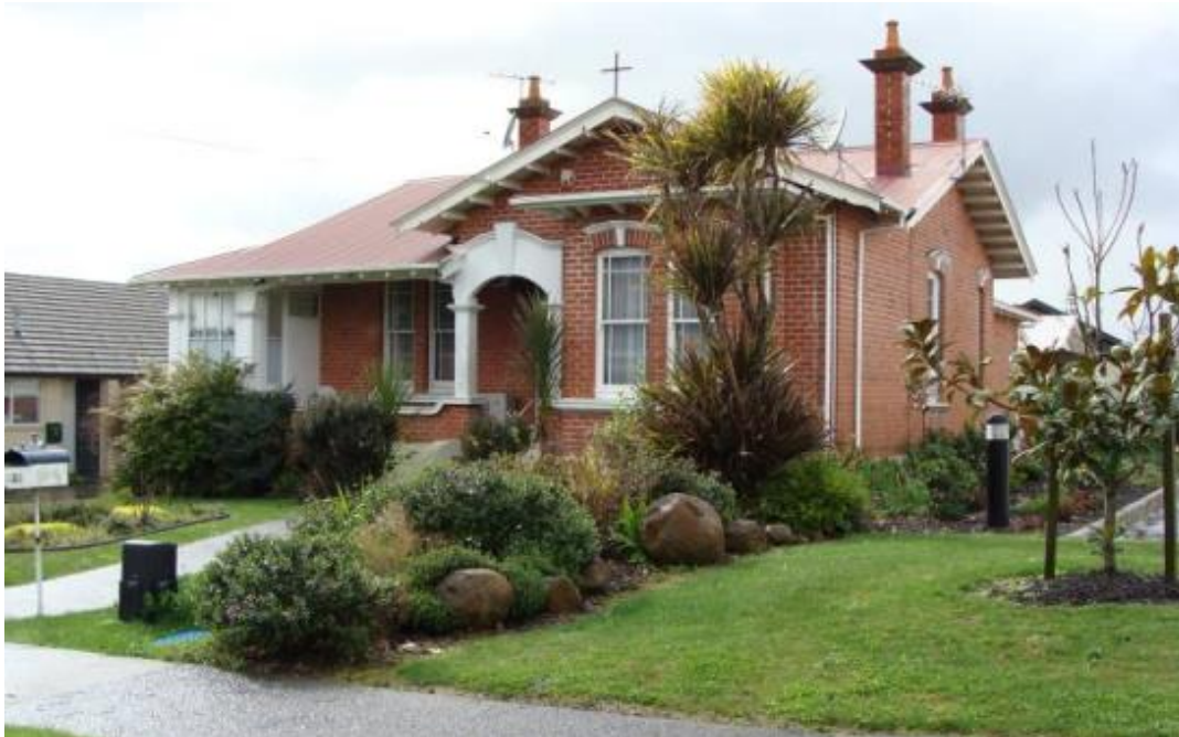
Figure 150. St Patrick's Presbytery, Seddon Street. Photo: AC, January 2014.
