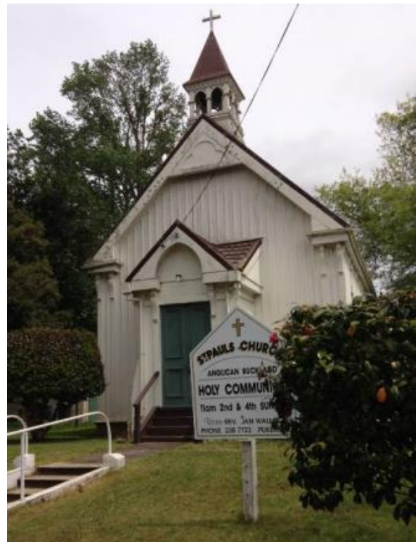
St Paul's Anglican Church front elevation. Photo: AC, January 2014.
