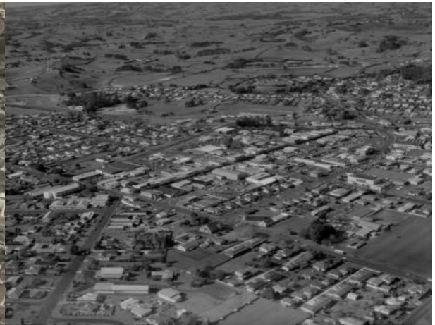
Figure 74. Aerial photograph of Pukekohe 1983. ATL: WA-77137-F.
