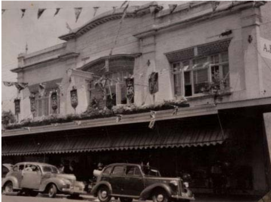
Figure 106. Beatty and Marshalls building, 30 December, 1953. Footprints 03971. Franklin Heritage Collection Pukekohe Library, Auckland Libraries.
