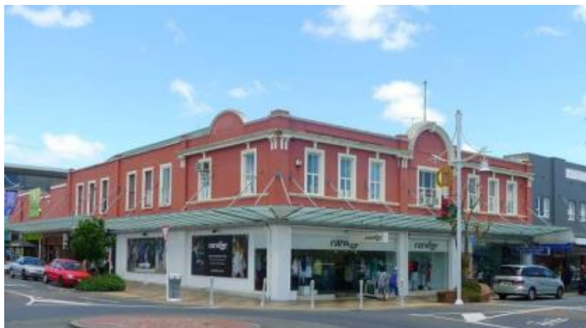
Figure 95. The Cooper & Curd building today. Photo: AC, 2014.
