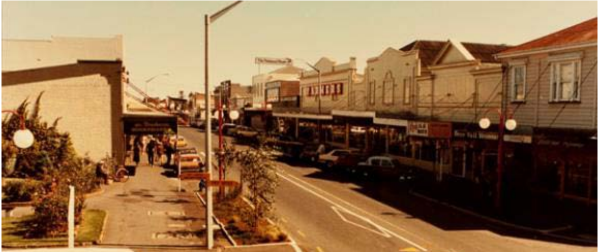
Figure 112. King Street, taken from intersection with Roulston Street. 1983, South Auckland Research Centre, FRA: I, 5 / Footprints 04860 (cropped).
