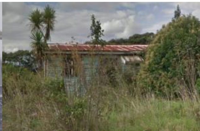
Figure 124. A farming building on Calcutta Road, Pukekohe which may have been used by Indian market gardeners which remains (but appears unused) today. Google street view 2009.
