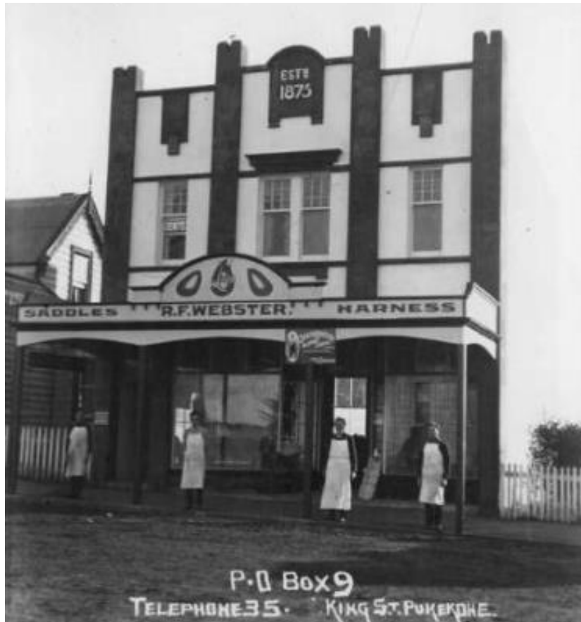
Figure 98. Former Webster building, King Street. Auckland Museum neg. PH NEG B400. DU436.136 P97b env1. Beattie, William.
