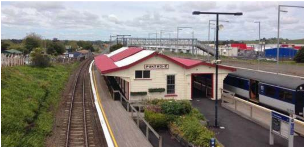
Figure 43. Pukekohe railway station as seen from pedestrian overbridge. Photo: AC, November 2013.
