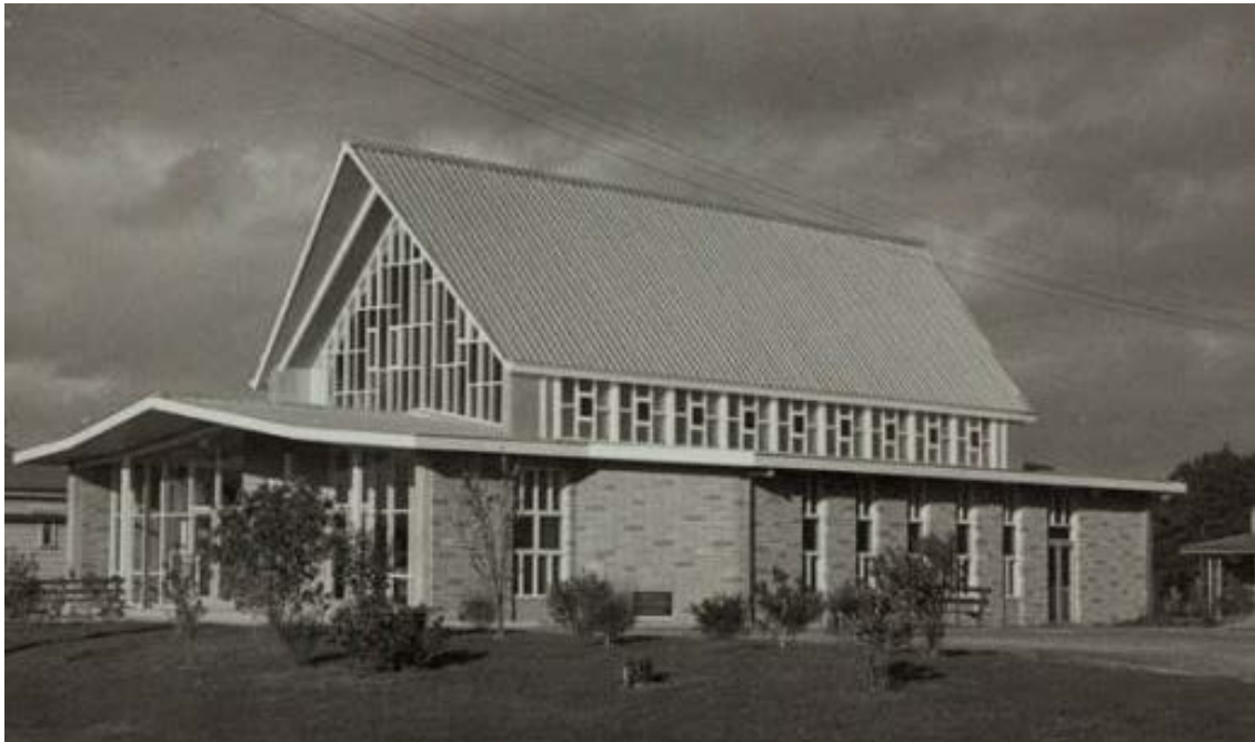
Figure 145. St James' Presbyterian Church -1962. FRA: I, 5 / Footprints 04880. Franklin Heritage Collection Pukekohe Library, Auckland Libraries.
