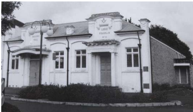
Figure 176. Masonic Hall in Pukekohe prior to demolition. Franklin Historical Society archives.
