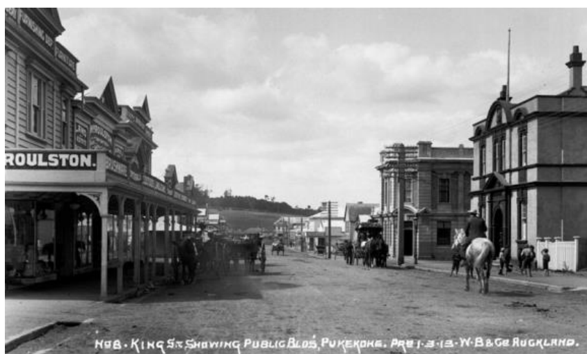
Figure 39. Road surface of the main street (King Street) of Pukekohe- images looking in opposite directions - then and now. Image titled: No. 8 King St showing public buildings, Pukekohe. Pre 1.3.13 W B & Co Auckland.
