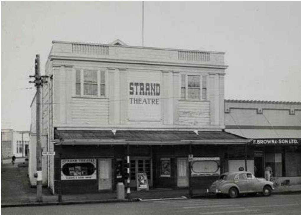
Figure 174. Strand Theatre, Pukekohe, c. 1956 FRA: I, 5 / Footprints 03100. Franklin Heritage Collection Pukekohe Library, Auckland Libraries.
