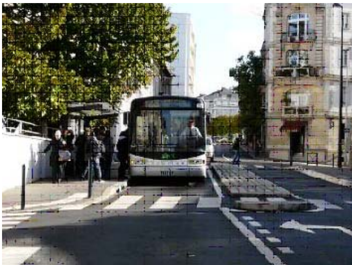
Figure 8. Traffic calming bus station / crossroads treated as roundabout
